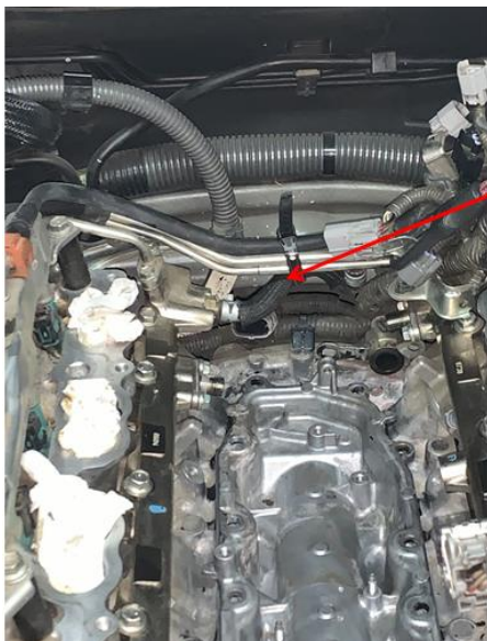
Supporting Rear fuel low pressure line
